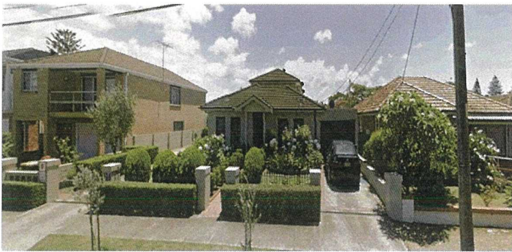
Single-storey dwelling at 126 Barton St, Image: Googlemaps
