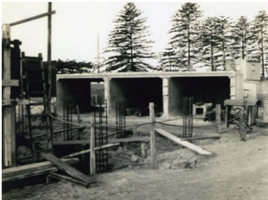
Figure 8 - Work underway on the building of the triple sewer at Kyeemagh after the reclamation and diversion of the Cooks River, late 1940s (Source: Bayside Library)
